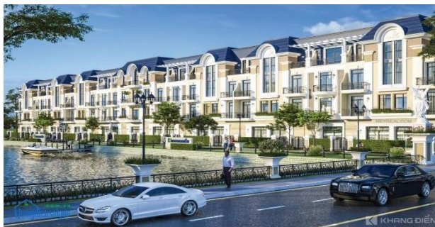
Figure 9: The Solina Project
